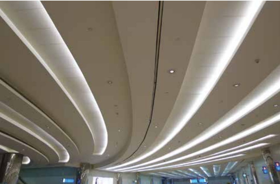
Suspended ceiling with SLAT™ (Self Levelling Access Trim) the unique patented Coopers' system
